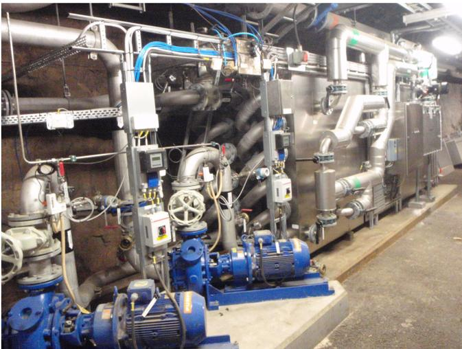
Figure 4. Two new tube heat exchangers installed in parallel below one of the anaerobic digesters, photo by Ulf Jansson, BYAK AB.
