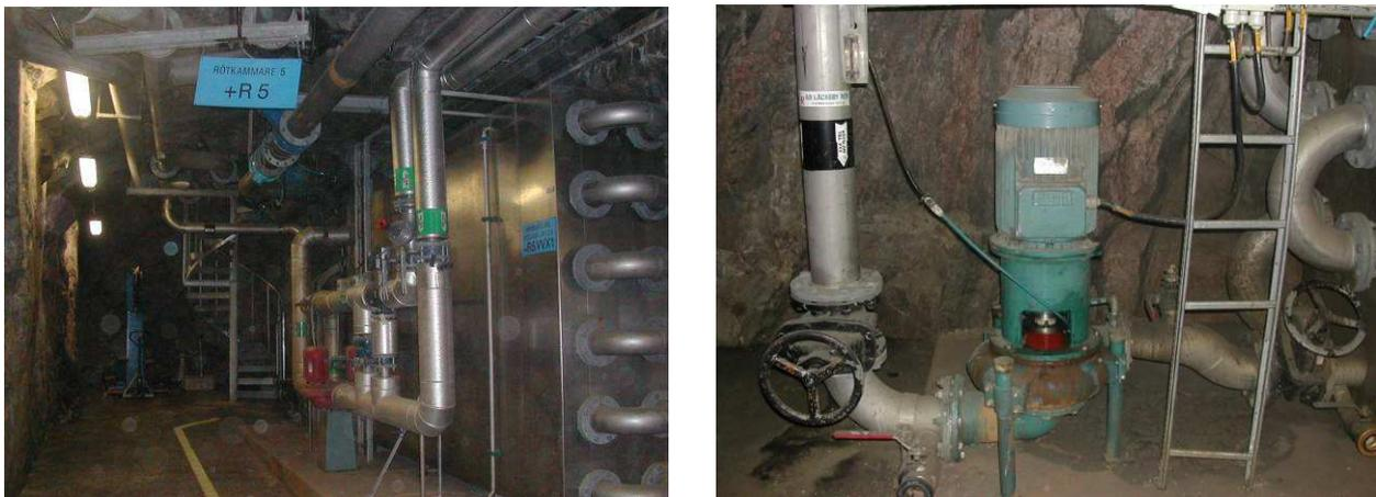
**Figure 7. On the left – the heat exchanger coil below anaerobic digester 5 at Henriksdal. On the right – the dosing point (at the bottom on the right) for the LiCl solution.**
