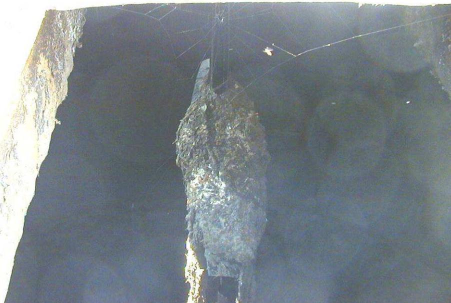
**Figure 25. The upper propeller blade is clogged with shreds.**
