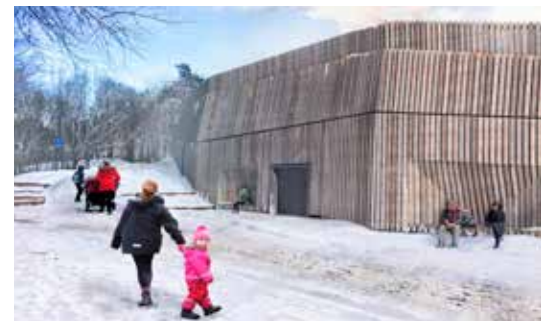
Stockholm Exergis pumpstation i Hammarbybacken Bild: Urban Design
